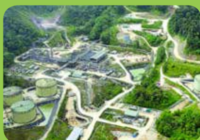
Kutubu Oil and Gas Production Operator: Oil Search Limited
