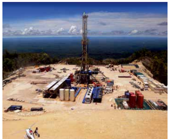
Drilling at Hides Gas field
