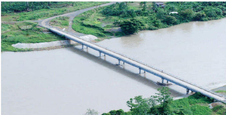
A bridge built in 2008 by Ramu Nico at a cost of K20 million has helped communities living between the Usino and Bundi areas of Madang Province access vital government services and transport their cash crops and garden produce to markets.
