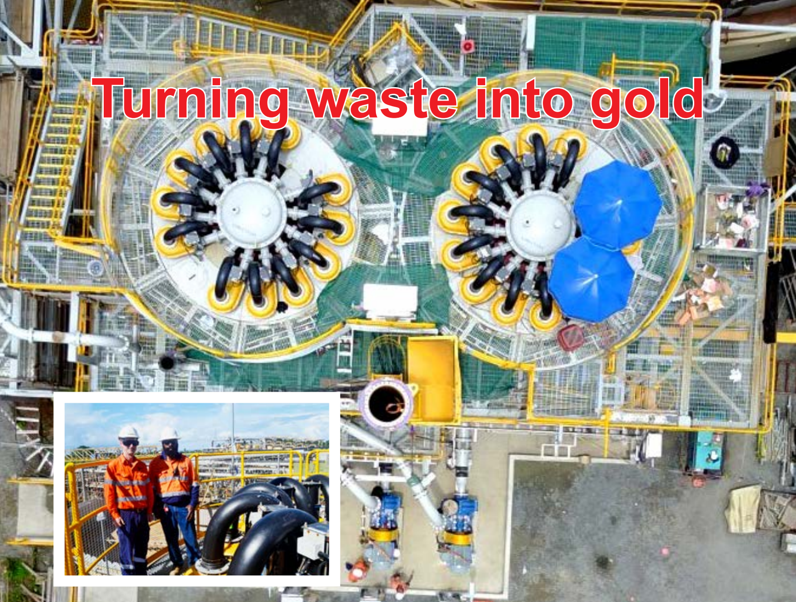
An aerial view of the Cyclone Tower at the Lihir mine, New Ireland Province. Insert: Newcrest Lihir's Engineering Projects Development department Andrew Moulds with Downer Construction Supervisor Richard Kuaru inspecting work at the top of the Cyclone tower. Pictures courtesy of Newcrest Mining
