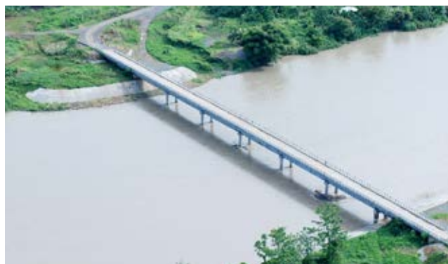
The bridge built by Ramu NiCo mine connecting Usino and Bundi in Madang Province.
